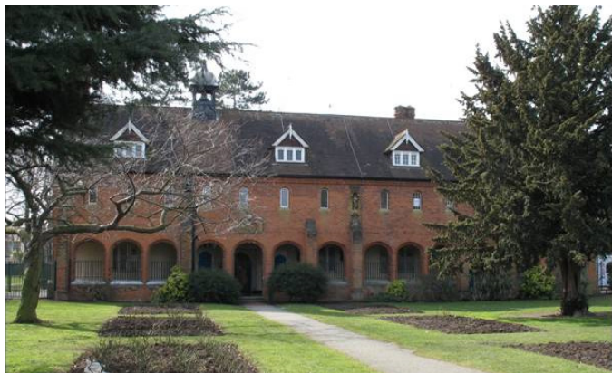
(Photograph taken prior to erection of hoarding around building for security)
